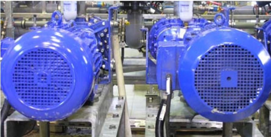
Self-ventilated motors for pump applications
