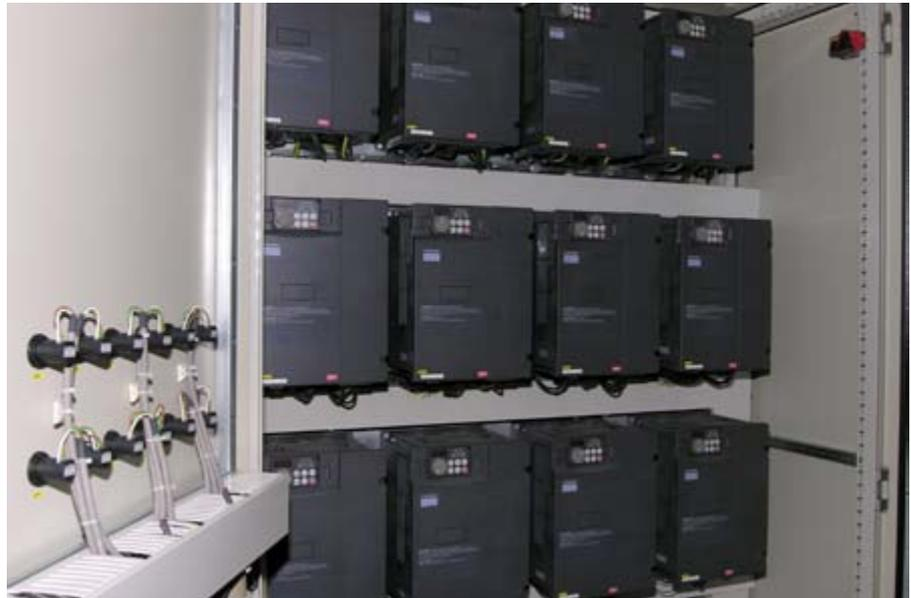
Inverters mounted in an electrical cabinet
